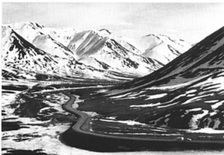
Figure 2. Spring break-up along the Dalton Highway and Trans-Alaska pipeline, in the Central Foothills region, Brooks Range, Alaska.
