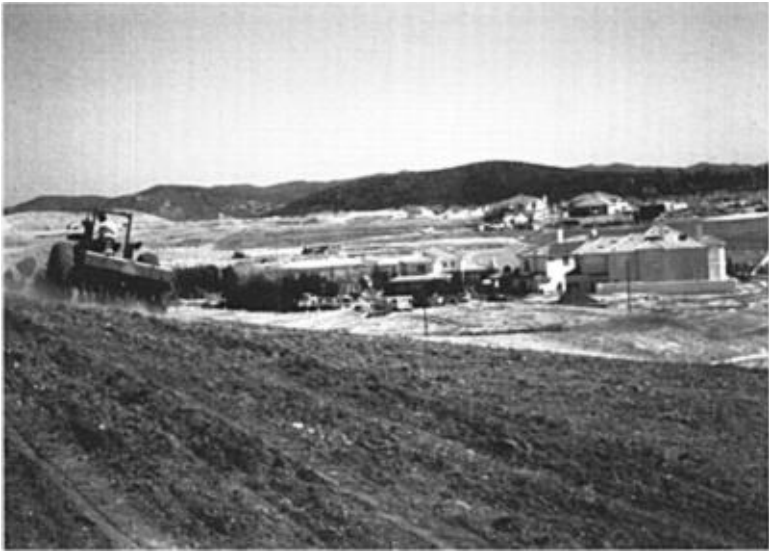
Figure 2. Drilling seed following site preparation, March 1991. View to the east.
